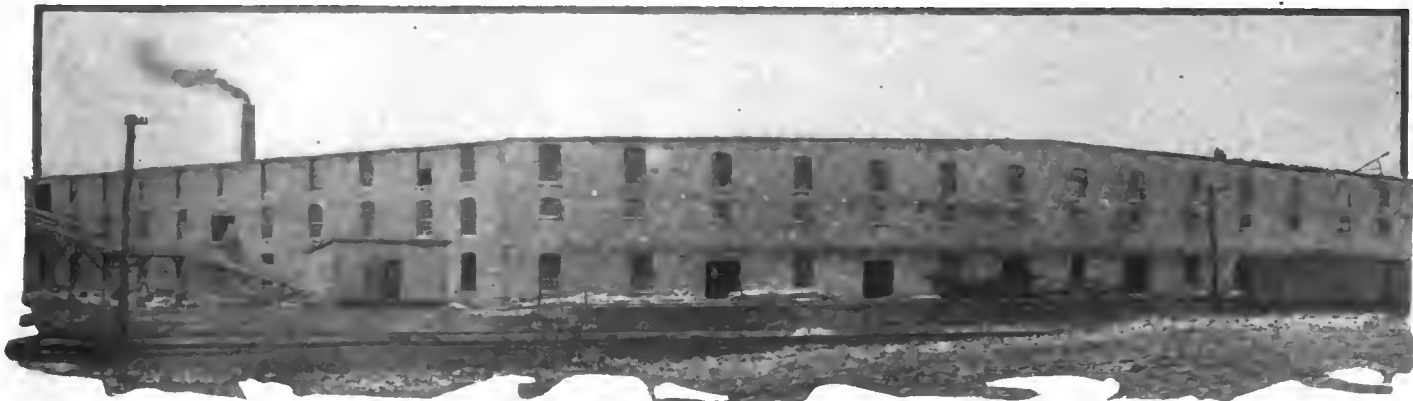
Three-story shipping and assembly plant of the Reo Motor Car Co., Lansing, Mich. This building was completed December 2, 1912. It is 252 by 252 feet, with 190,512 square feet of floorspace and a capacity of 1,600 cars. The floors are of cement. The building is equipped with an automatic sprinkling system and is connected with the other parts of the plant by an overhead runway. Its covered platform accommodates twenty 40-foot box cars, thus making the loading capacity 120 cars per day.
